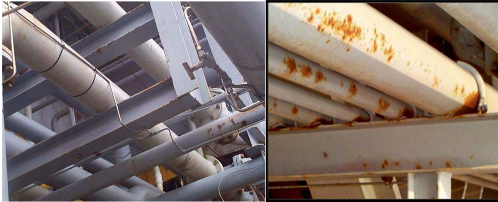
Fig 1.5 U-Bolt Stabilized Beam Supports.
